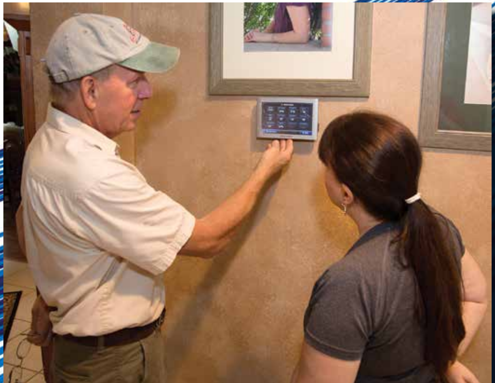
Efficient Climate Control owner Paul Stamper explains the workings of the control panel to a homeowner.
